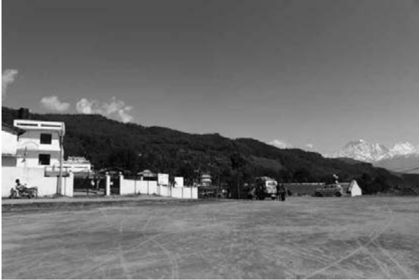
Figure 2 District administration office, Charikot, Dolakha district
